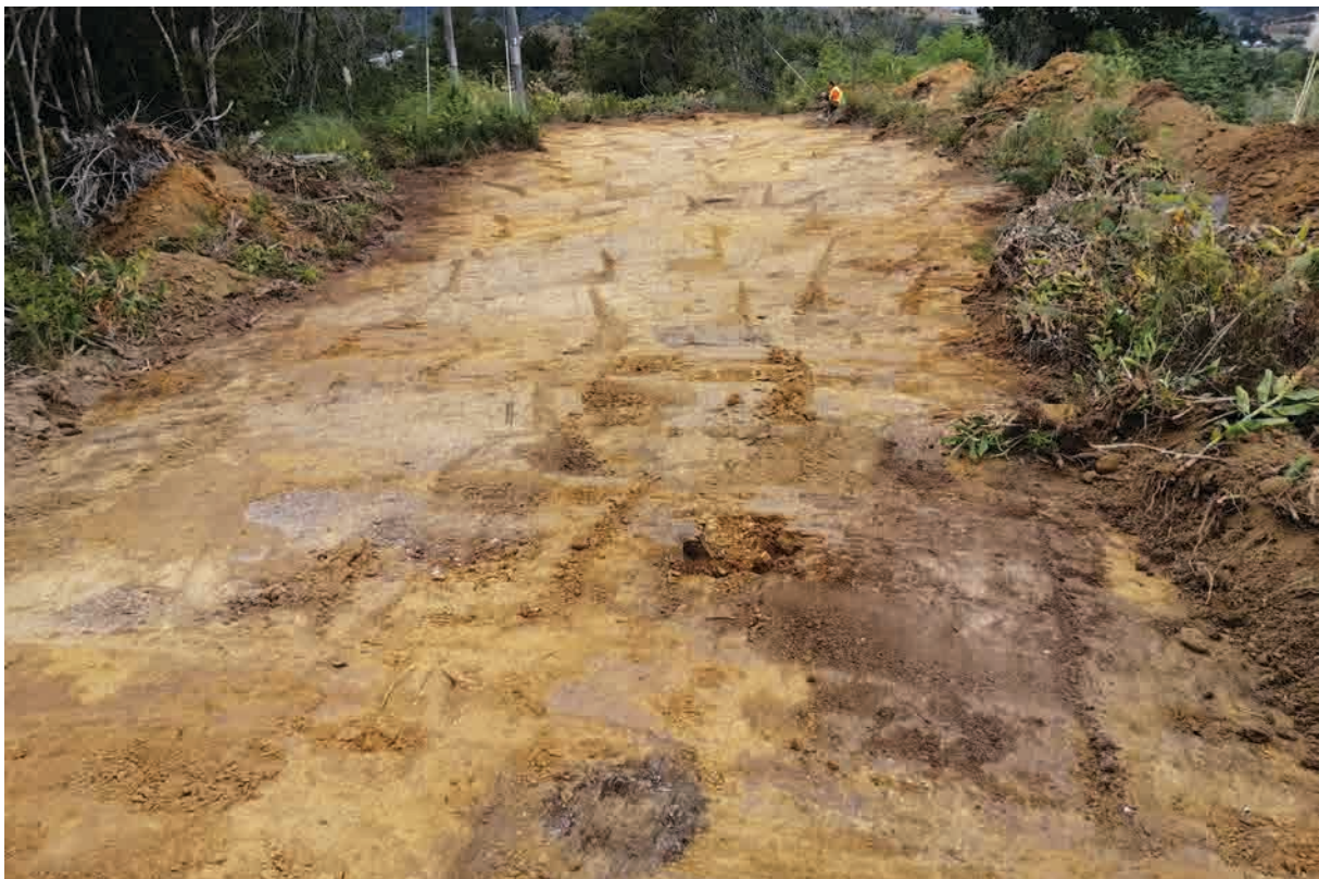
Figure 7. Area B terrace after topsoil stripping
